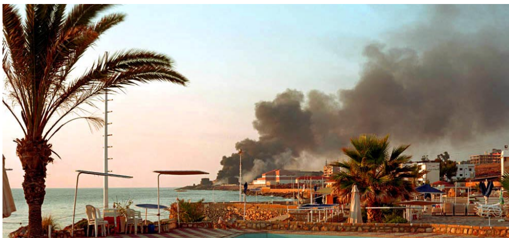
An oil Fired power Station in Jiyeh.
