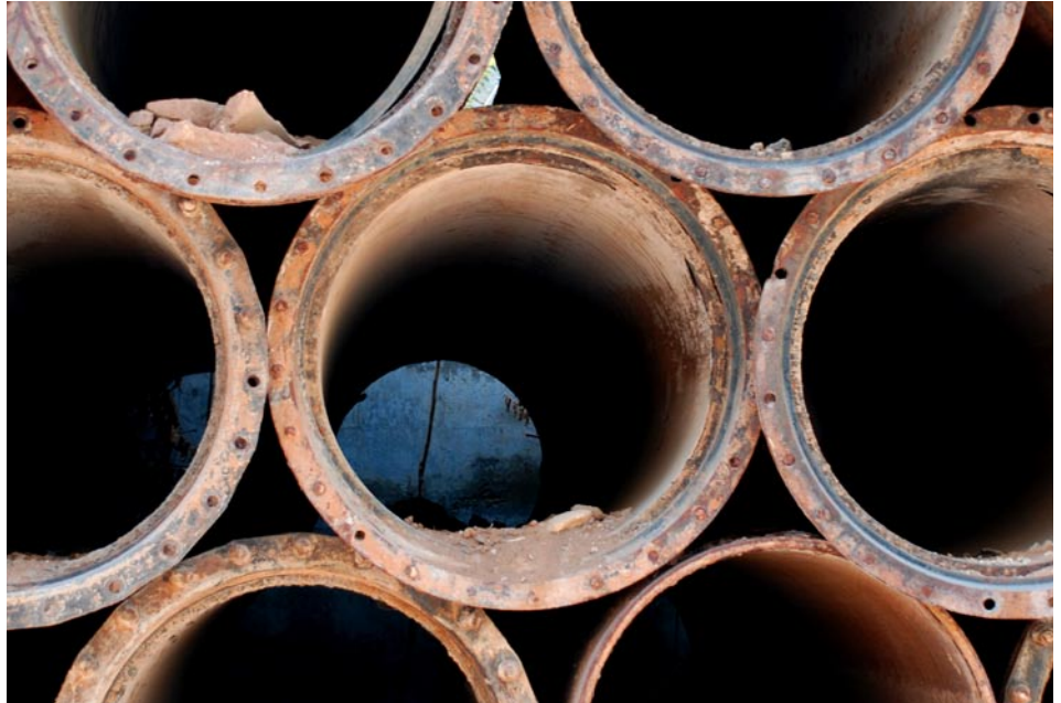
Rusted water pipes.
