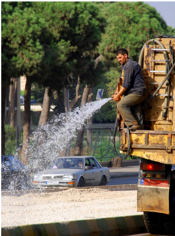
Roadworks in Beirut
