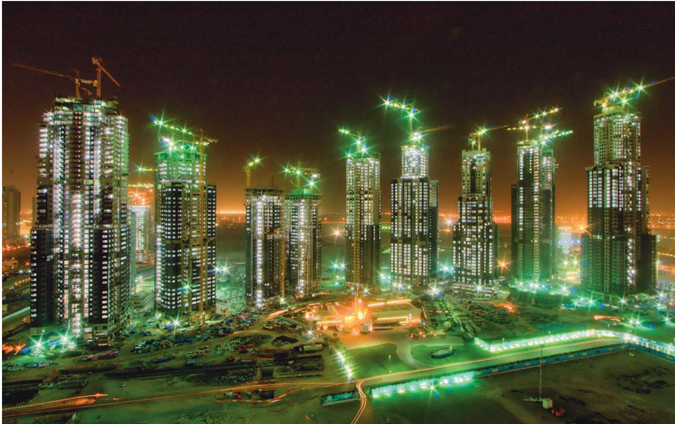
One of the many construction projects in Dubai.
