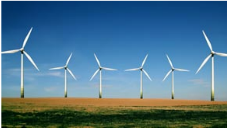
Wind turbines – a clean form of energy.
